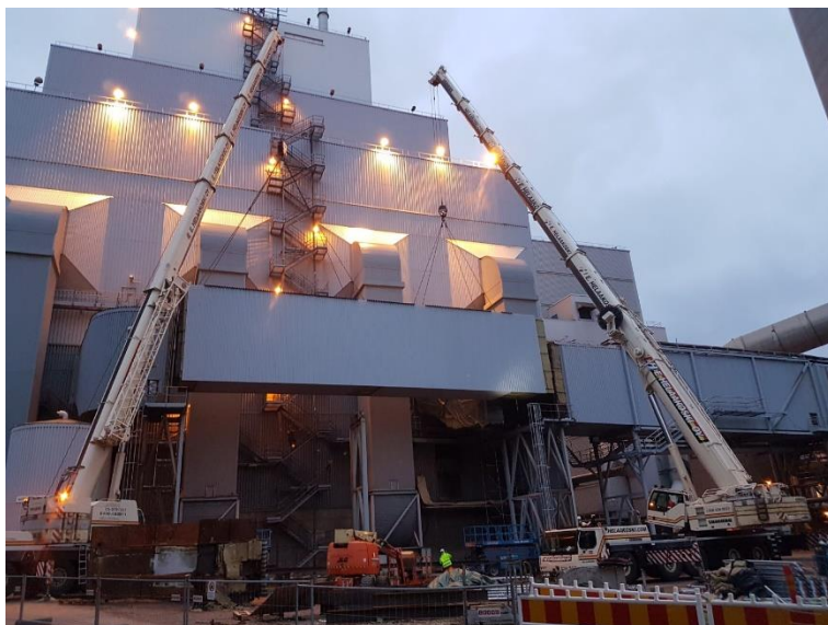
Final ESP duct lifting at the Stora Enso Imatra plant (courtesy from Stora Enso)
